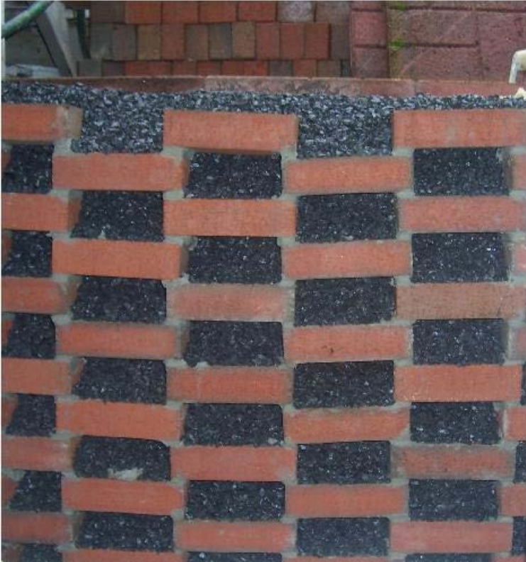
Particular Wall™ made of Bricks
